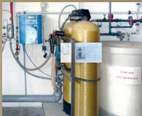
TTC's osmosis system decalcifies the cleaning water
